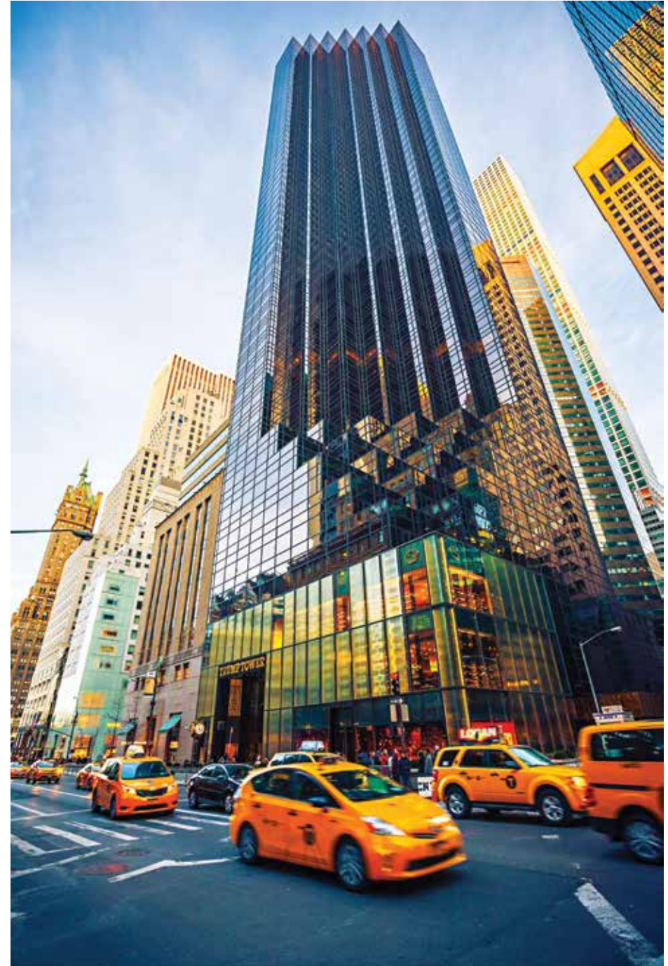
A view of the unusual sawtooth set-back feature of Trump Tower's upper floors, a feature that impressed architecture critics.
